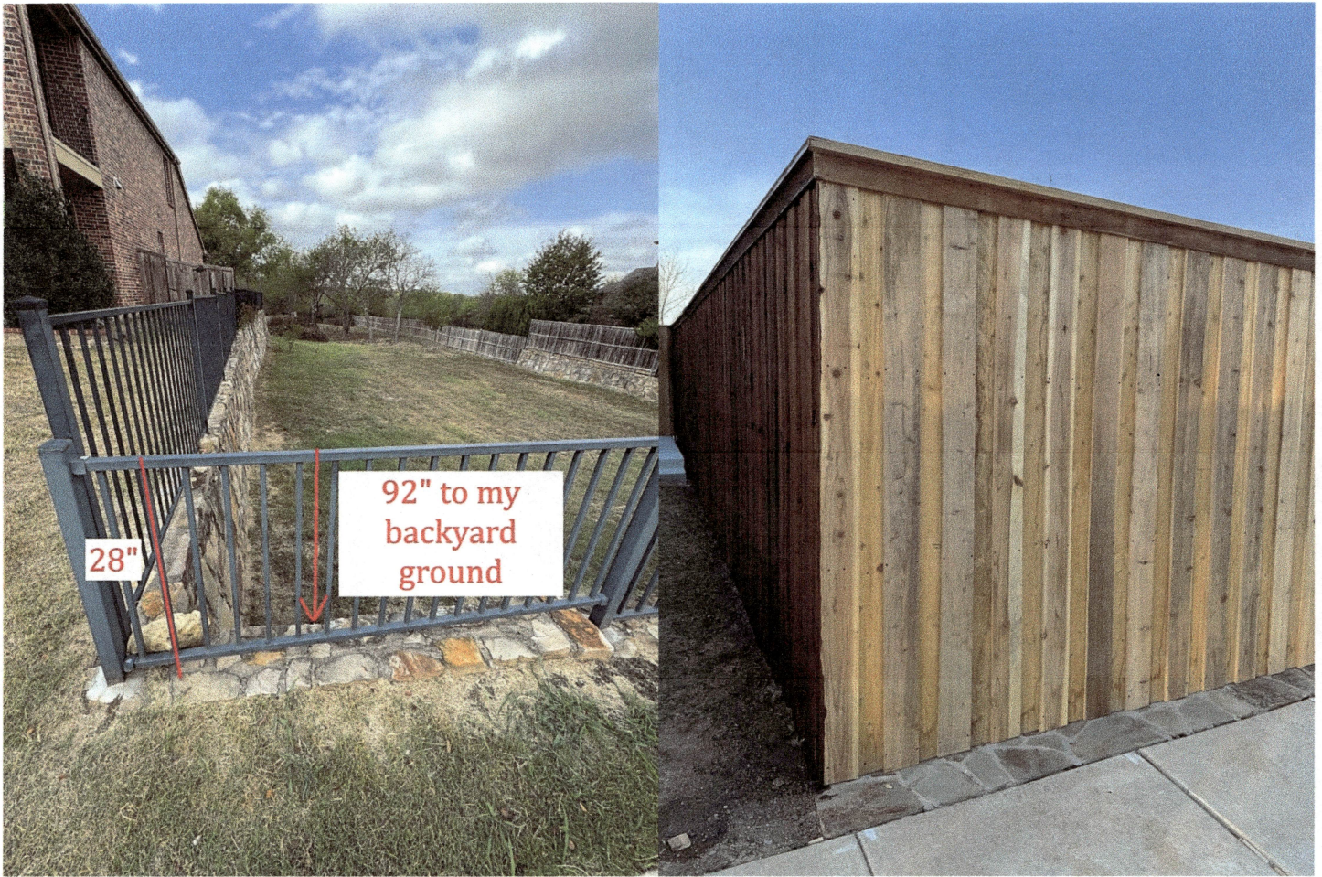
Figure 3. 1111 Bentley Drive Before and After Looking North (mid-staining)
