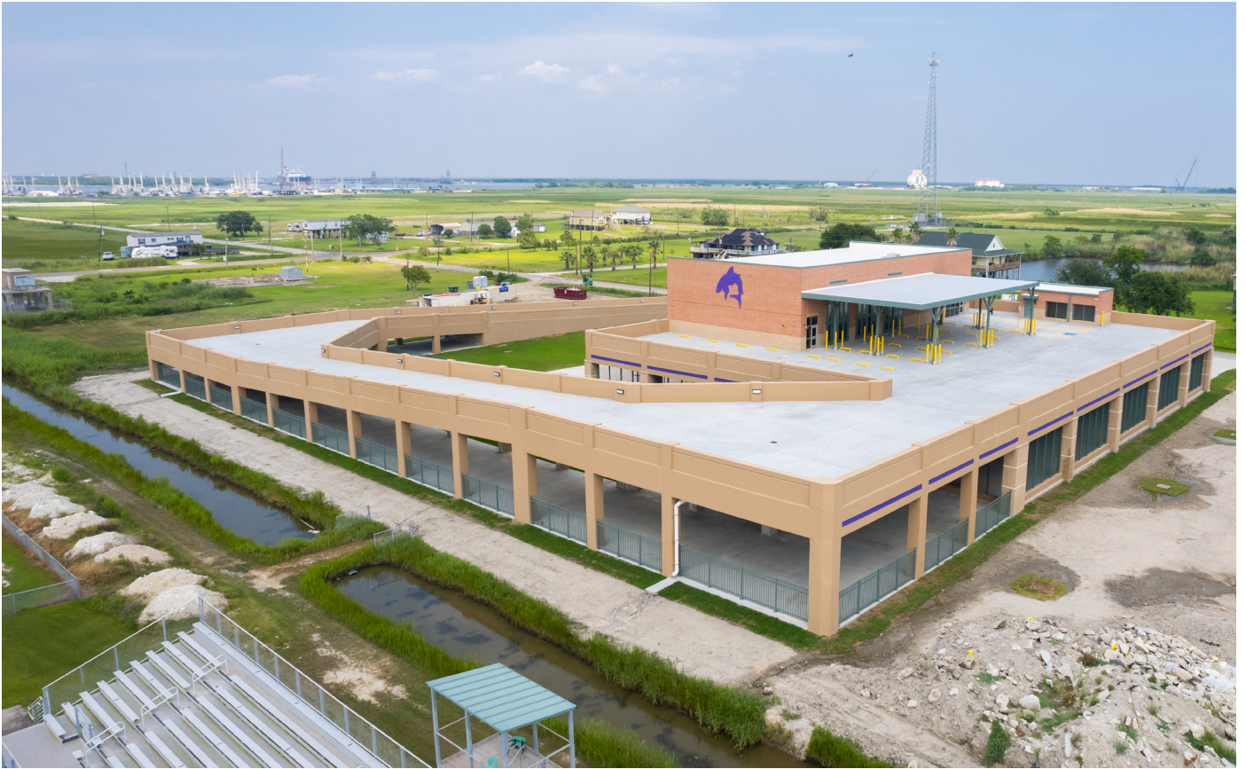
Sabine Pass ISD, Transportation Center/Parking Garage
