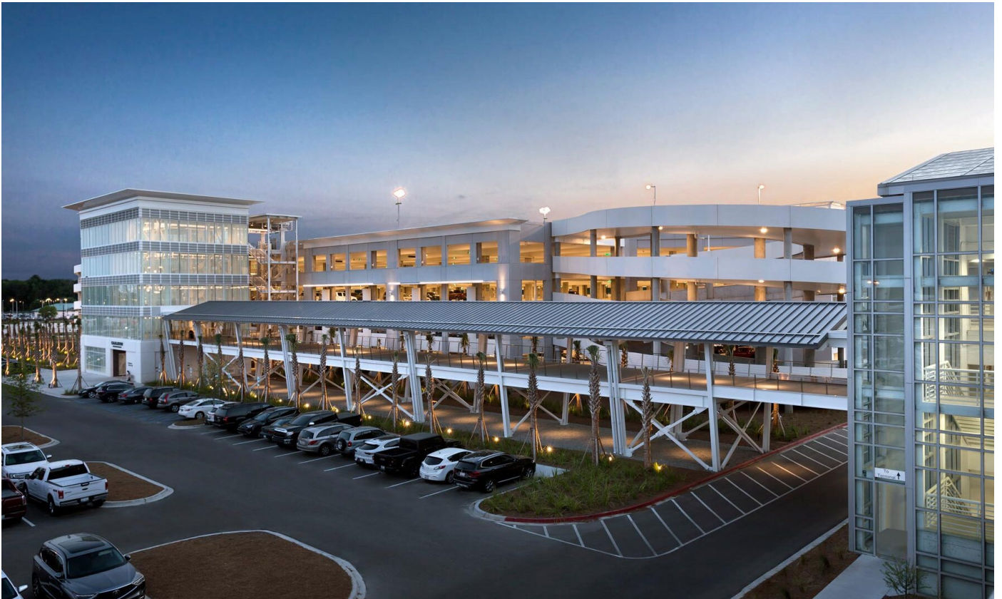
Charleston Airport Parking Garage *Services provided by parent company, Cumming Group
